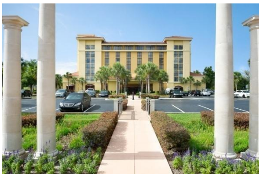
EMBASSY SUITES ORLANDO NORTH
